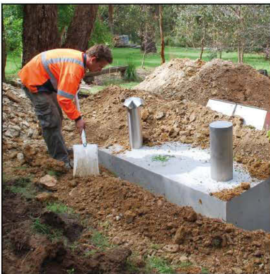
Compacting by hand.
